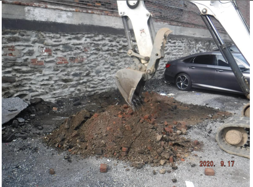
Photo 1 – Excavation of TP-3, facing southwest.
