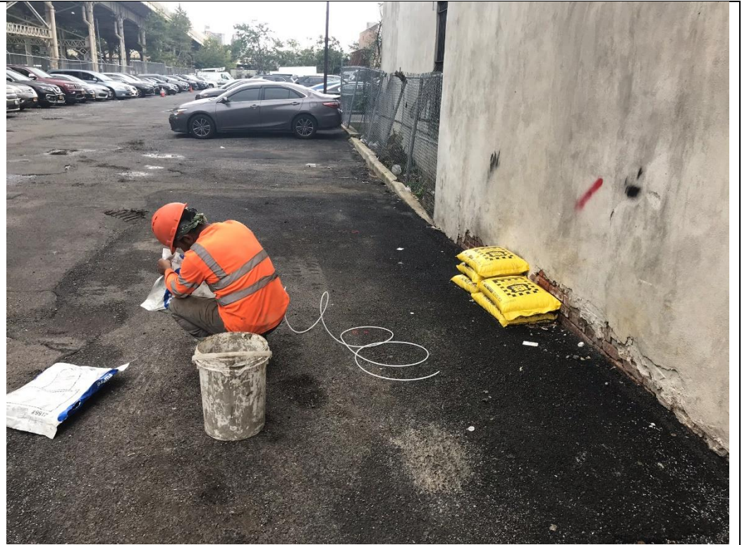
Photo 3 – AARCO installing LSV-14, facing east.
