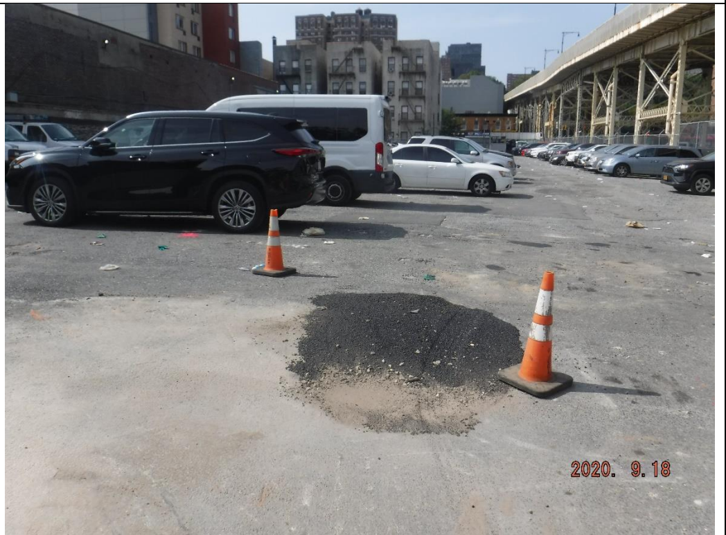
Photo 2 – Surface restoration of TP-2 with cold patch asphalt, facing west.
