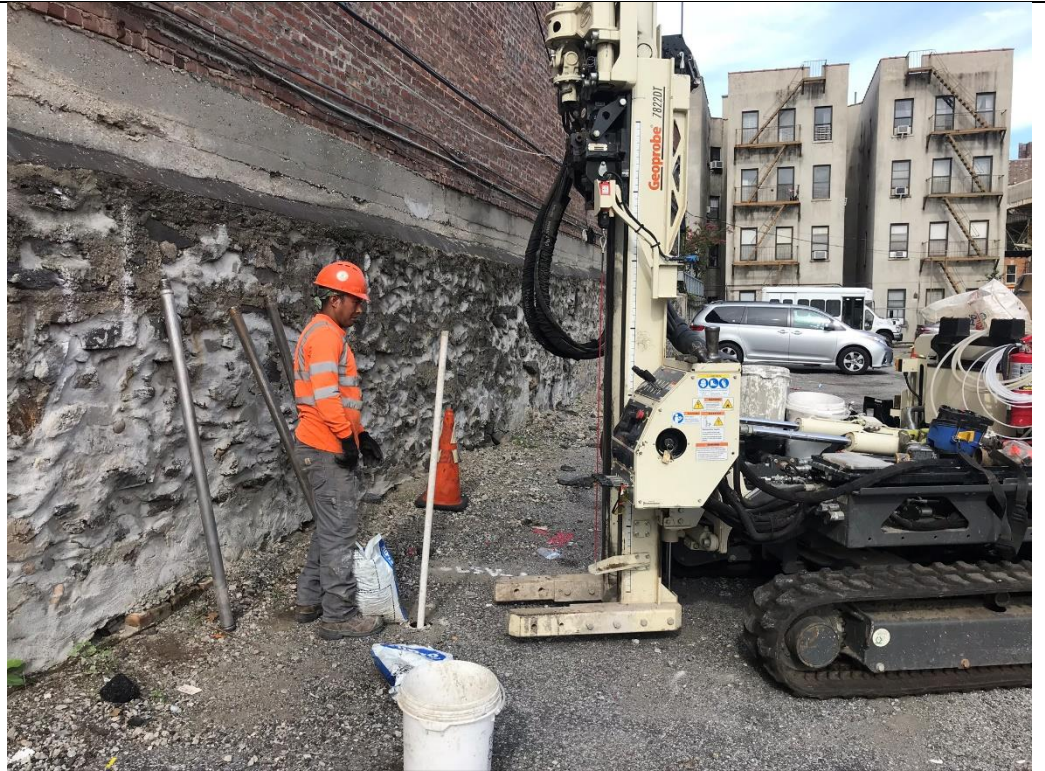
Photo 1 – AARCO installing LSV-16, facing west.
