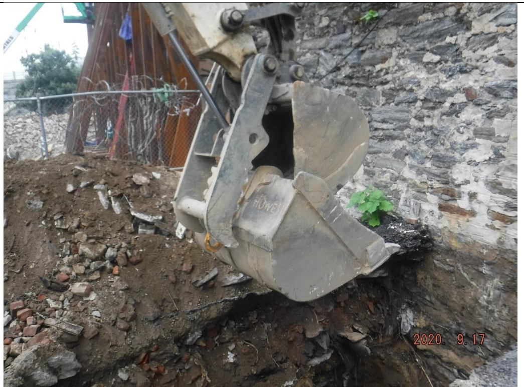
Photo 2 – Excavation of TP-4, facing south.
