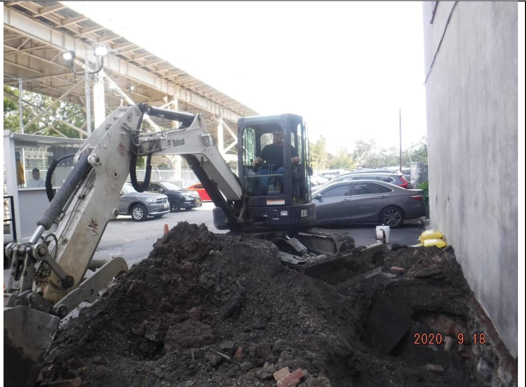
Photo 1 – Excavation of TP-1, facing east.
