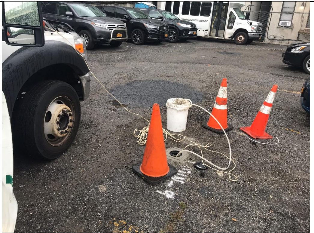
Photo 2 – Well development of LMW-9, facing southeast.
