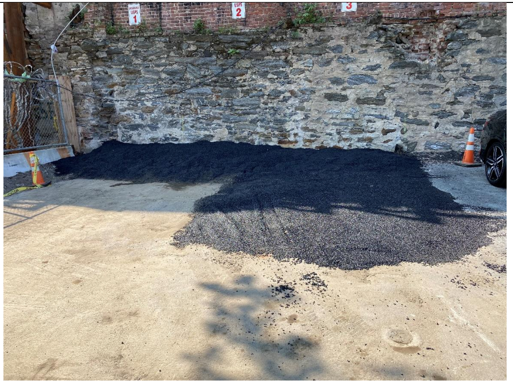
Photo 2 – Excess test pit material covered with cold patch asphalt, facing south.
