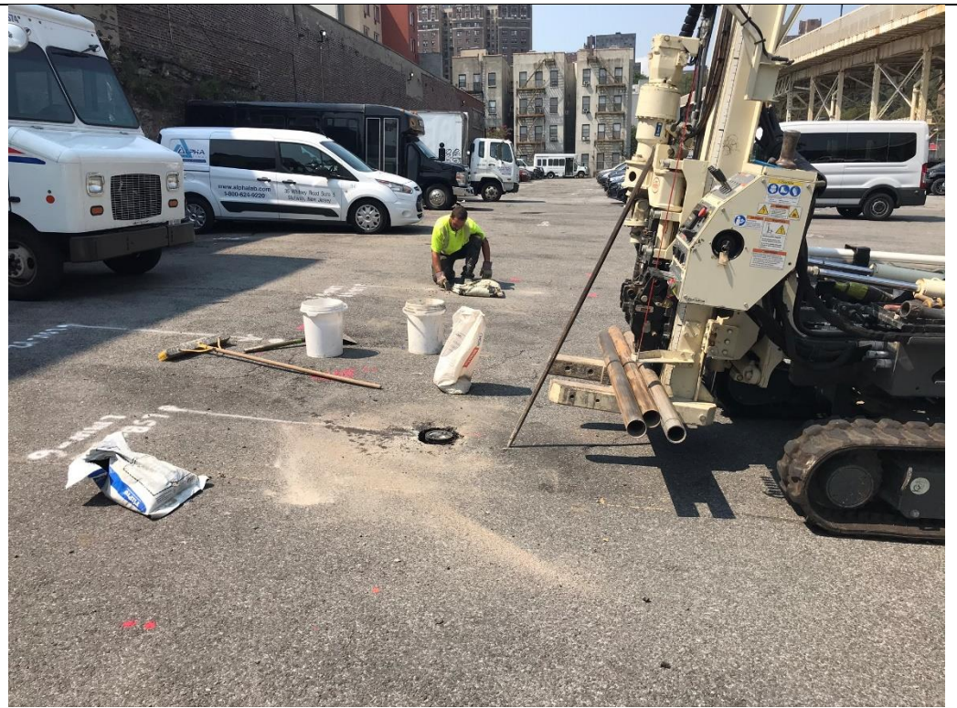
Photo 3 – Installation of manhole cover at LMW-6, facing southwest.
