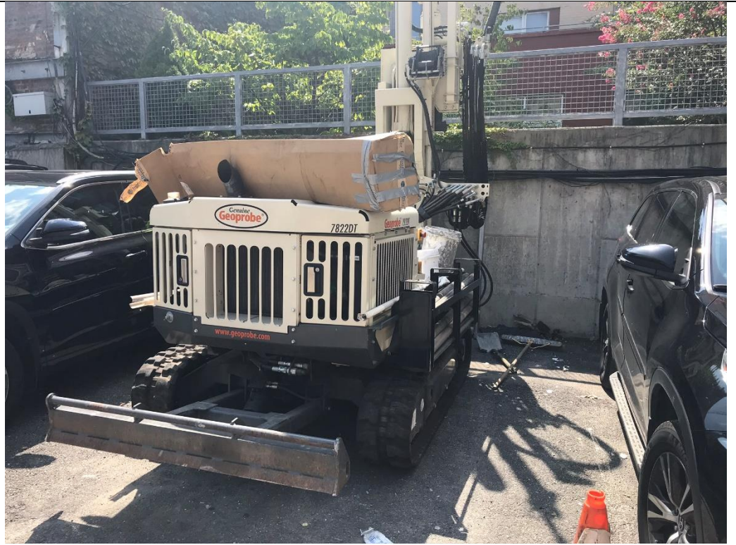
Photo 1 – AARCO drilling at LSV-15, facing southeast.
