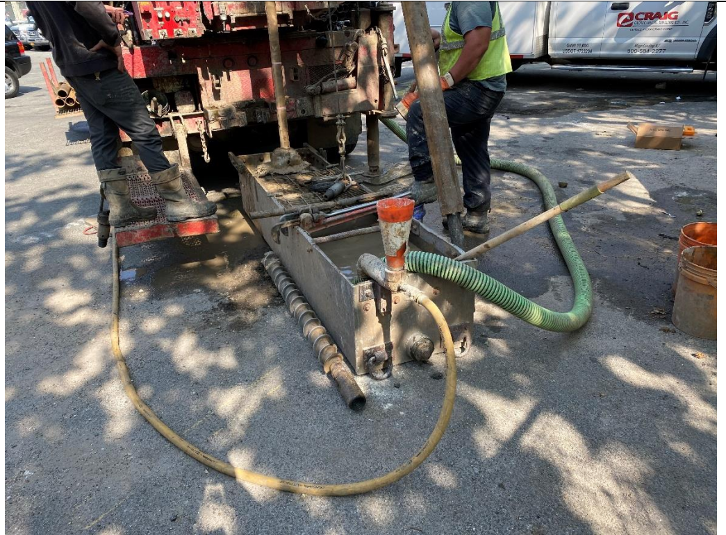
Photo 1 – Geotechnical drilling at LB-13, facing north.
