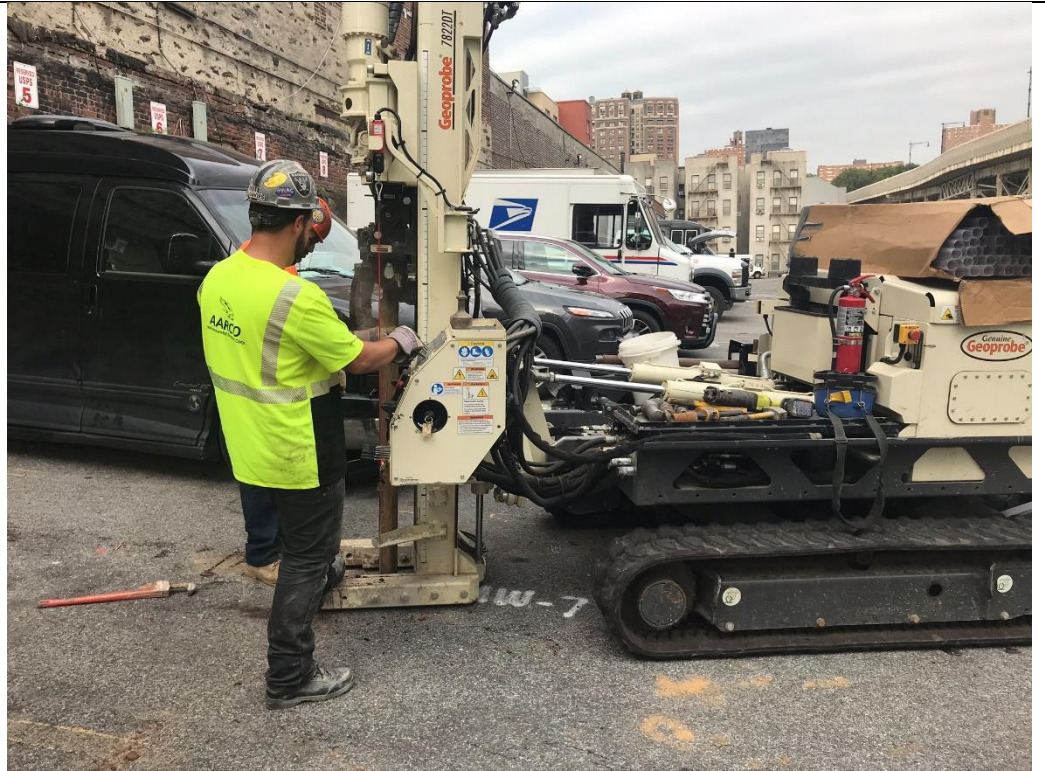
Photo 1 – AARCO installing LMW-7, facing southwest.
