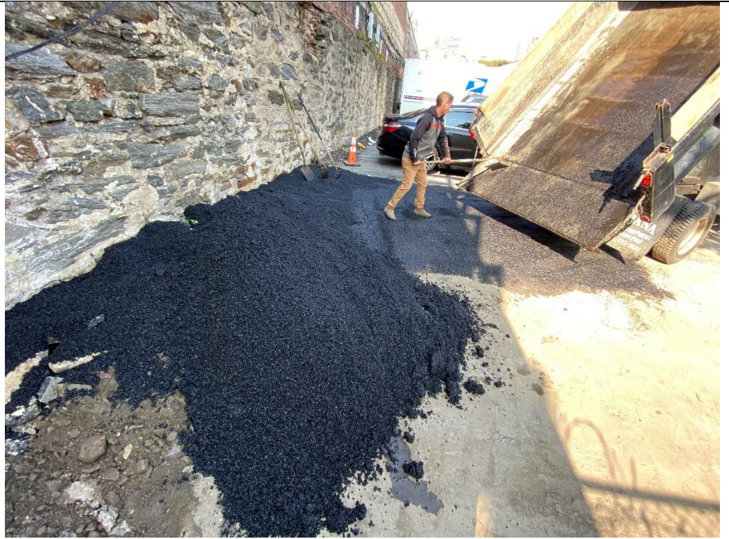
Photo 1 – Cold patch asphalt surface restoration, facing west.
