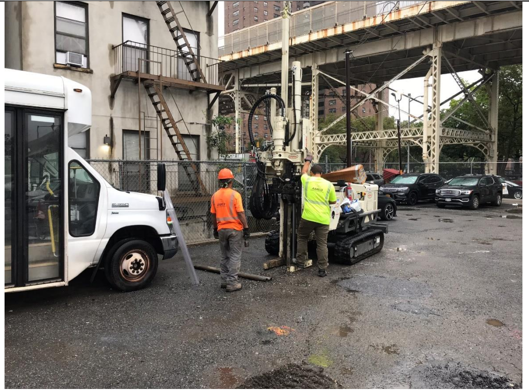
Photo 1 – AARCO drilling at LSB-57, facing north.
