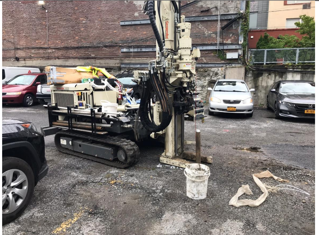
Photo 1 – AARCO installing LMW-9, facing southwest.
