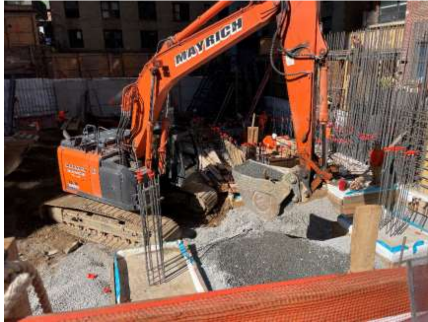
Photo 11: View of Mayrich removing 0.75-inch stone in the northwestern part of the site, facing south. Taken on 06/28/2022
