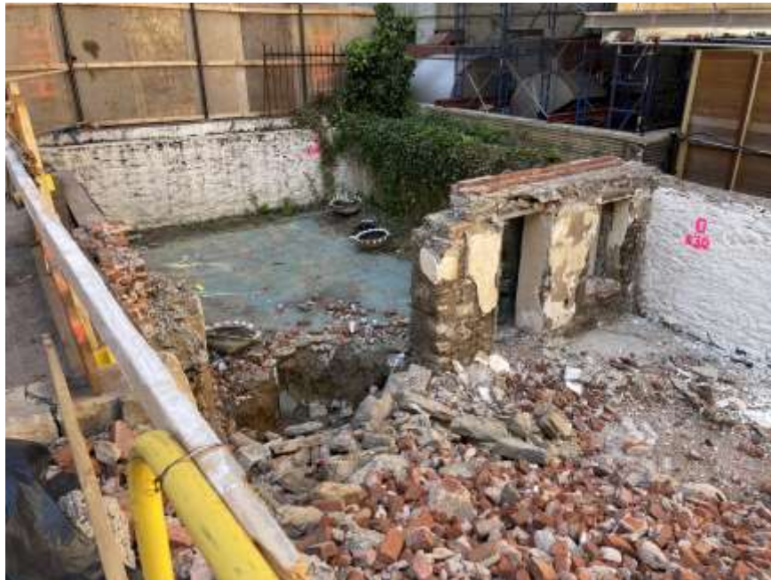
Photo 2: View of site prior to mobilization for excavation activities, facing south. Taken on 05/09/2022
