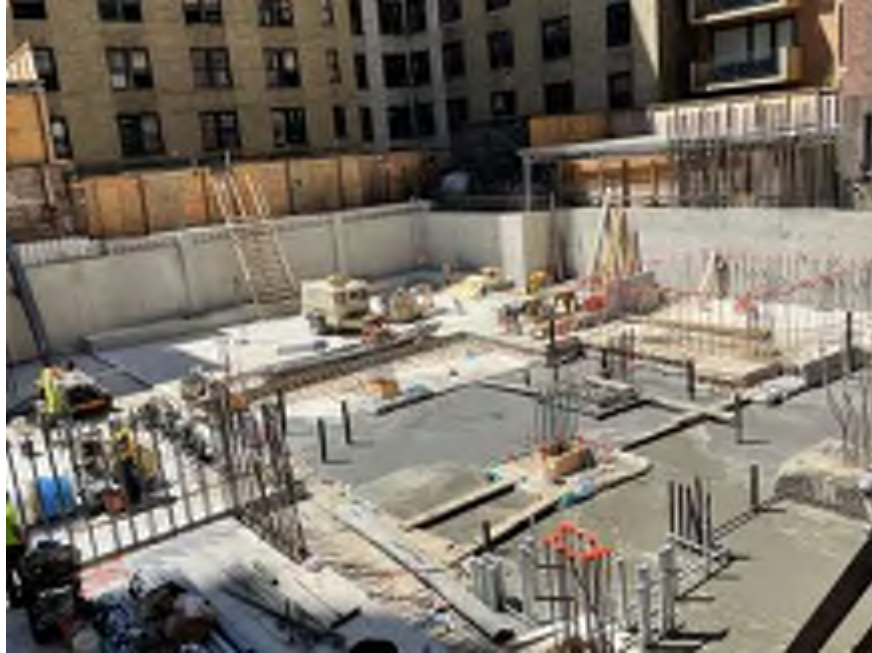
Photo 3: General view of the site (facing southwest). Taken 08/19/2022
