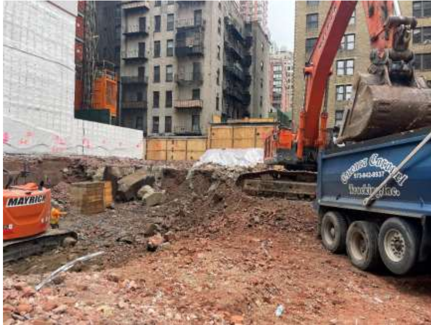
Photo 3: View of Mayrich Construction (Mayrich) loading a truck with construction and demolition (C&D) material for off-site disposal, facing southeast. Taken on 05/13/2022
