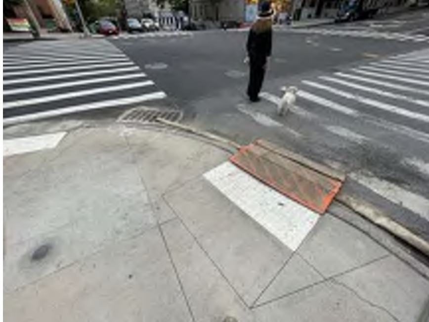
Photo 1: View of off-site components of the site's dewatering system on West End Avenue (facing northwest).
