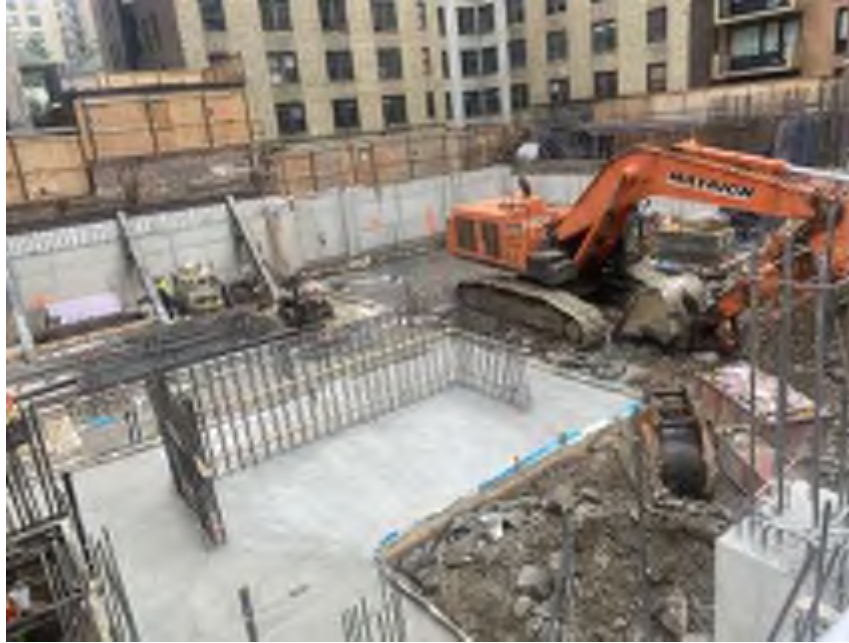
Photo 1: General site view of the site (facing southwest).
