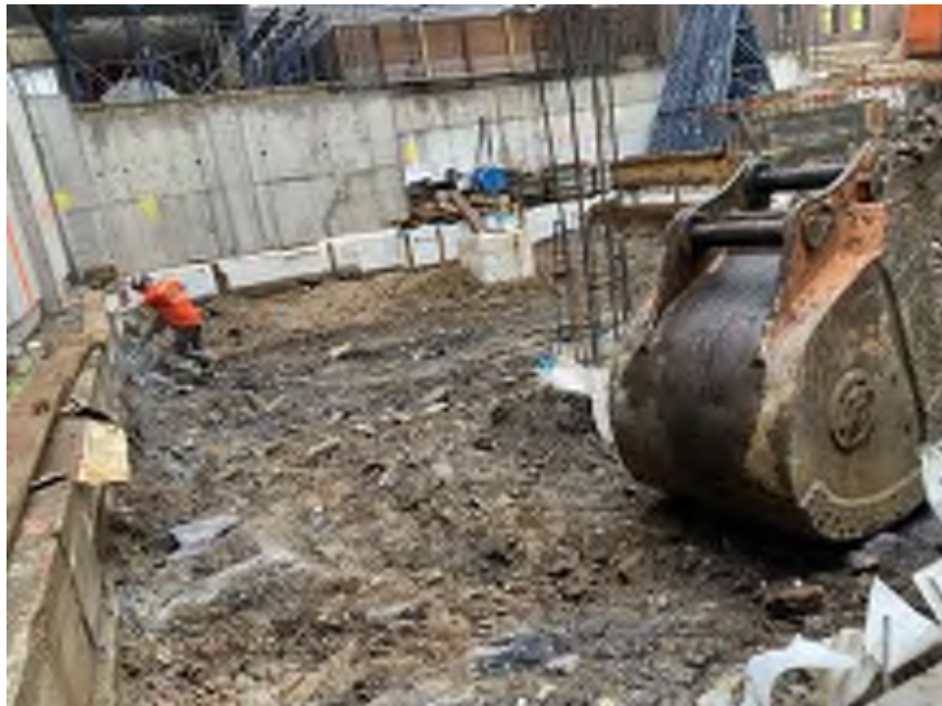
Photo 2: Mayrich chipping bedrock in the southwestern part of the site (facing east).
