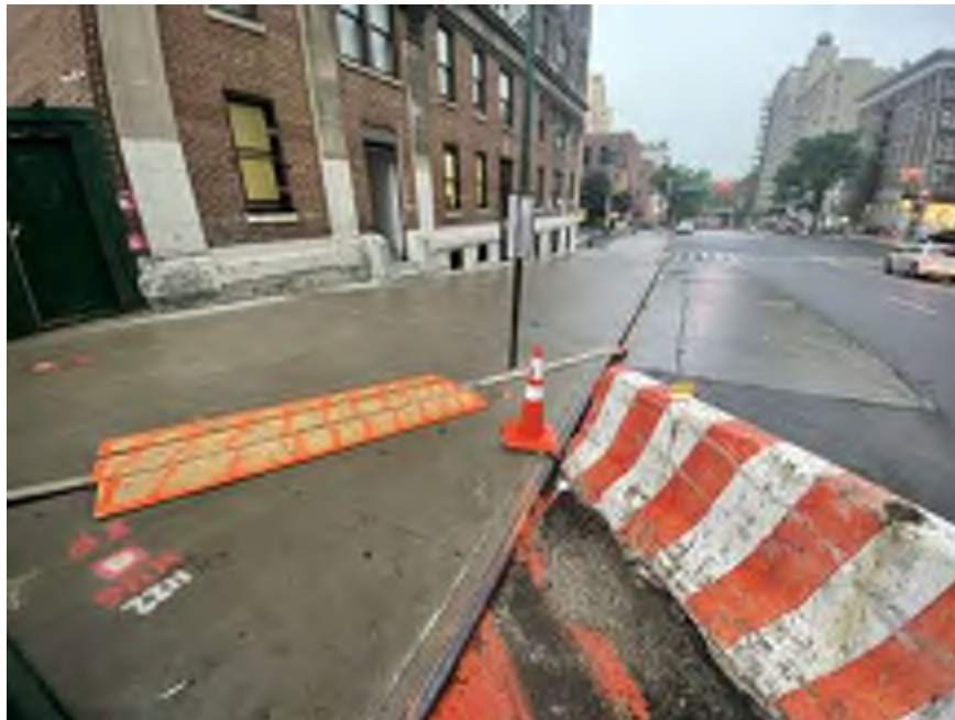
Photo 2: View of the off-site segment of the dewatering system (facing west).
