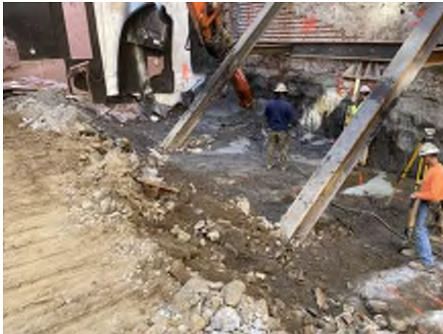
Photo 2: View of Mayrich using dust suppression during bedrock chipping on the western part of the site, facing southwest.
