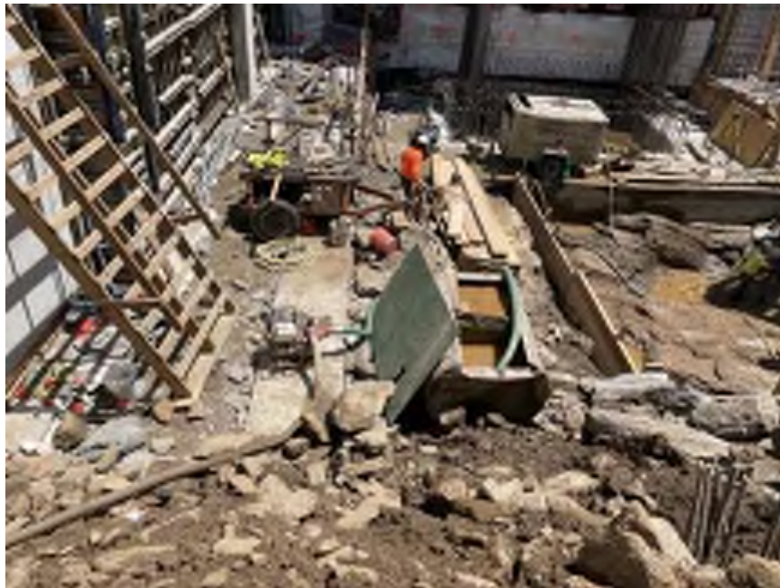
Photo 2: View of the on-site segment of the dewatering system (facing east).
