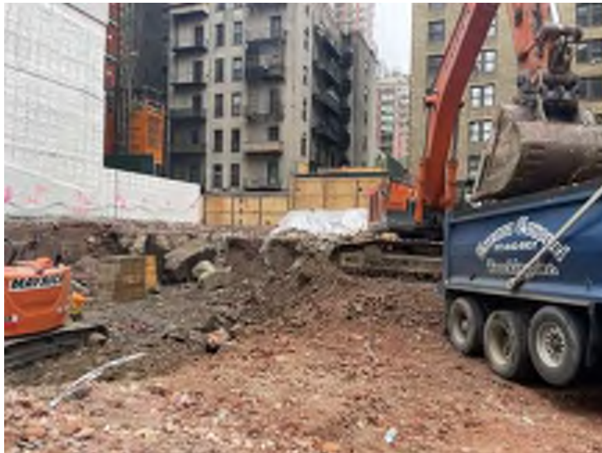
Photo 2: Mayrich applying dust suppression during export of C&D for off-site disposal (facing southeast)
