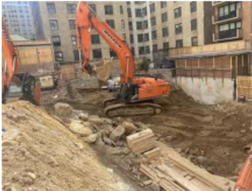
Photo 2: General view of the southwestern part of the site (facing south).
