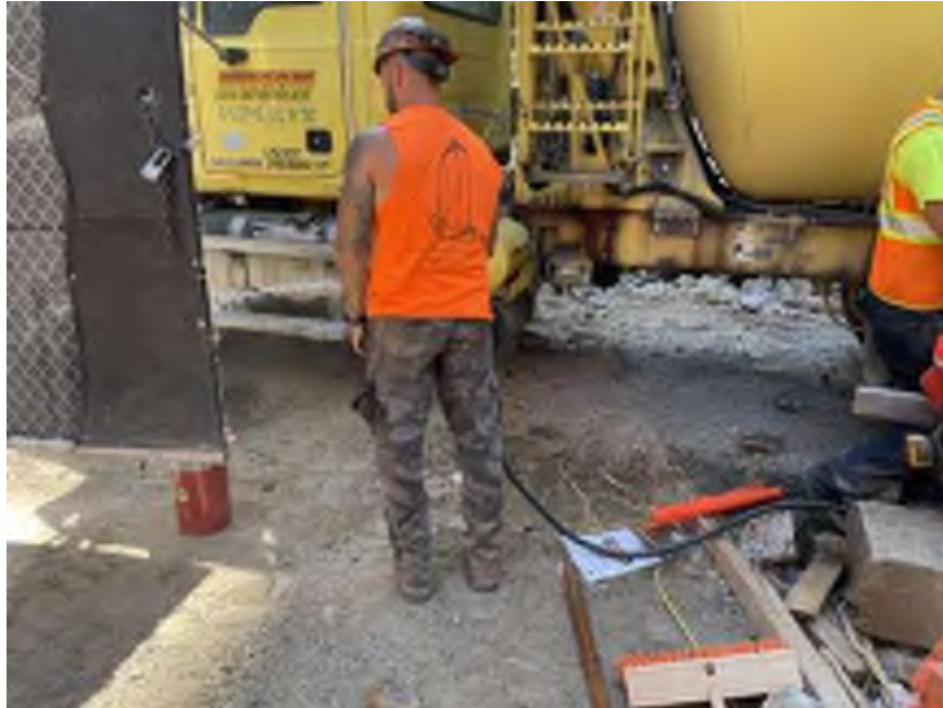
Photo 2: Mayrich using dust suppression on the trucking ramp (facing east).
