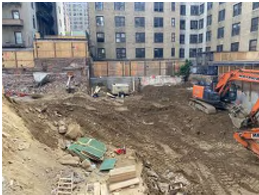
Photo 2: General site conditions at end of work day (facing south)
