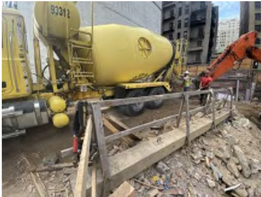
Photo 2: Mayrich cleaning tires of a concrete truck prior to the truck leaving the site (facing southeast).
