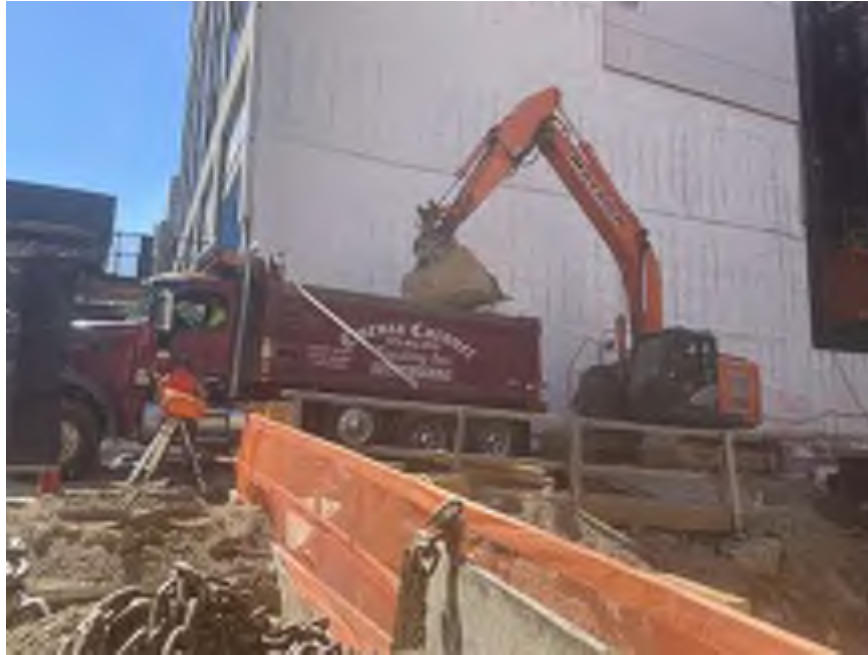
Photo 2: View of Mayrich exporting C&D debris for off-site disposal (facing east).
