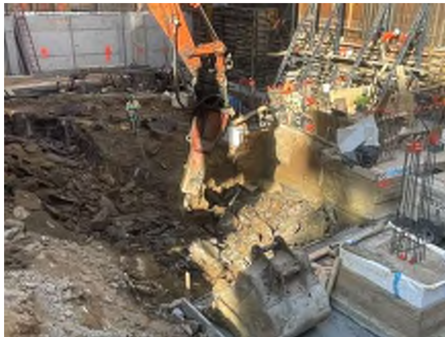
Photo 2: Mayrich using dust suppression while chipping bedrock in the central part of the site (facing east).
