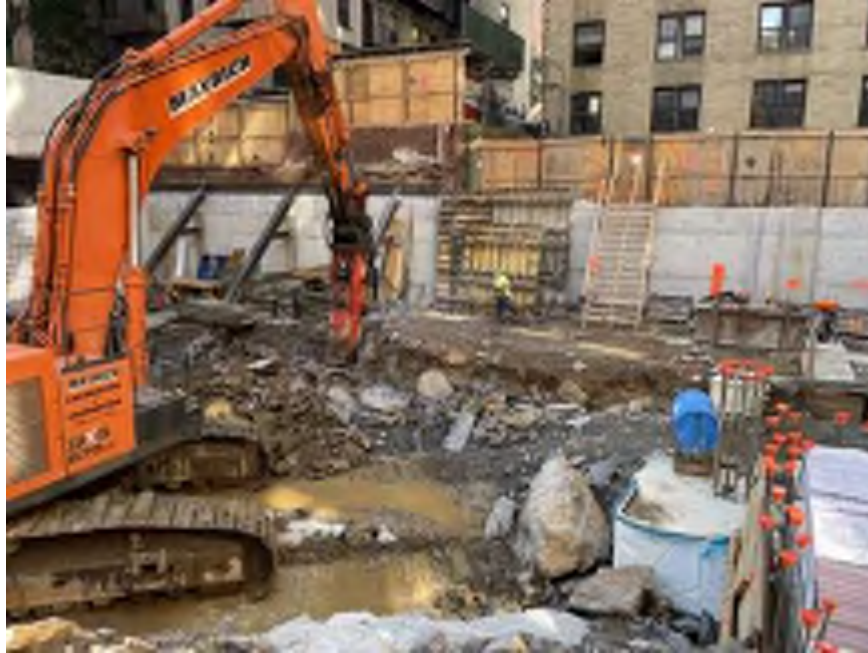
Photo 1: Mayrich using dust suppression during chipping of bedrock (facing south).
