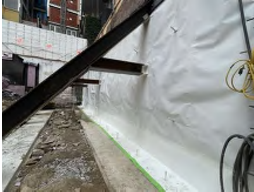
Photo 1: General view of waterproofing installed along southern site boundary (facing east).
