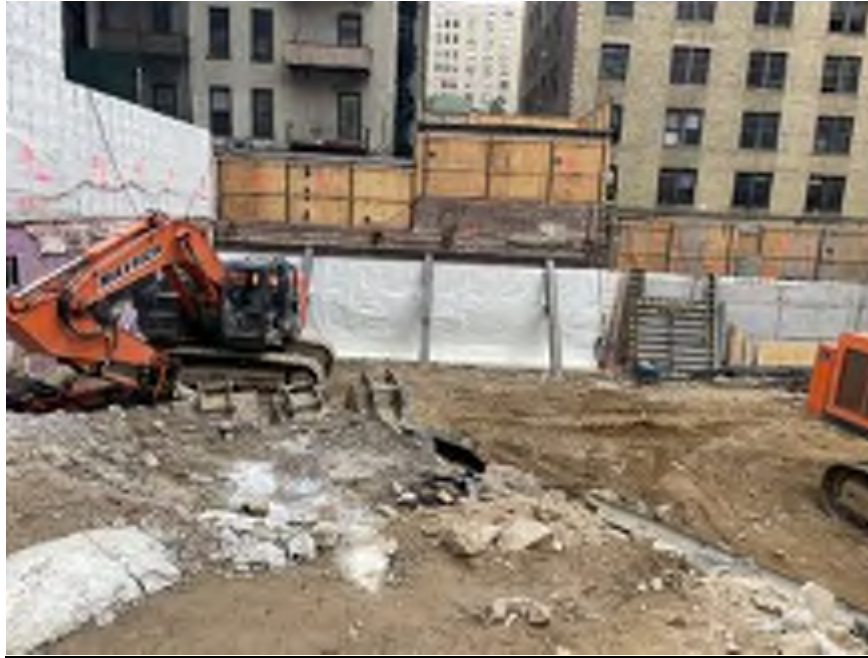
Photo 1: General view of the eastern part of the site (facing south).
