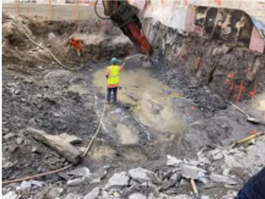
Photo 2: View of Mayrich using dust suppression while chipping bedrock in the northeastern part of the site (facing north).
