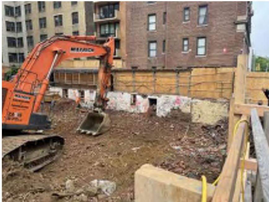
Photo 2: General view of the northwestern part of the site (facing west).
