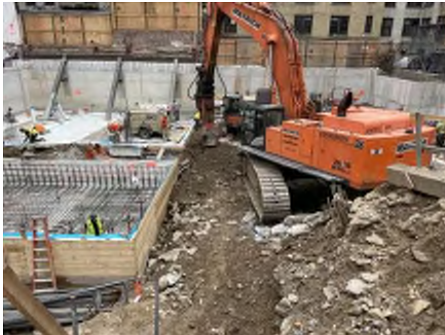
Photo 2: View of Mayrich chipping bedrock in the southern part of the site (facing south).
