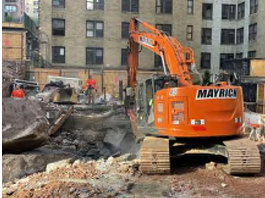
Photo 1: Mayrich applying dust suppression while chipping concrete (facing south).
