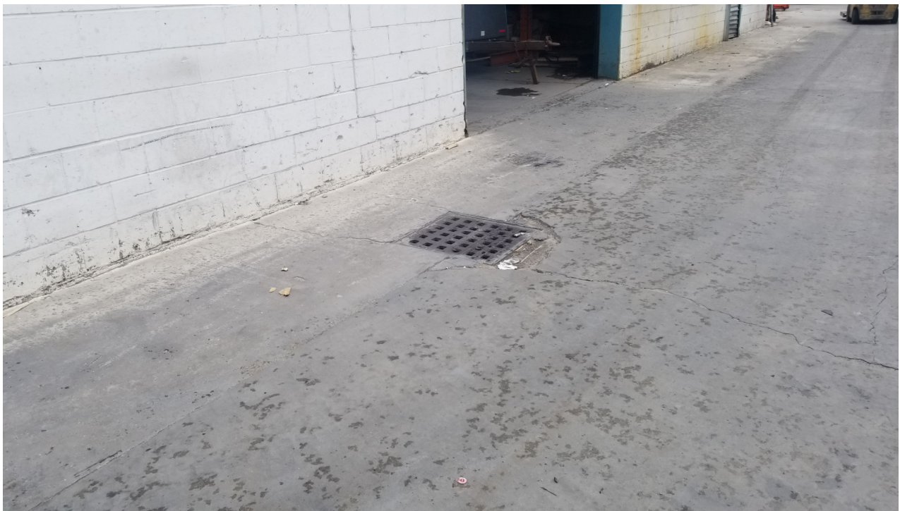
Photograph 10: View of stormwater inlet in concrete parking area along 135 th Street, facing north.
