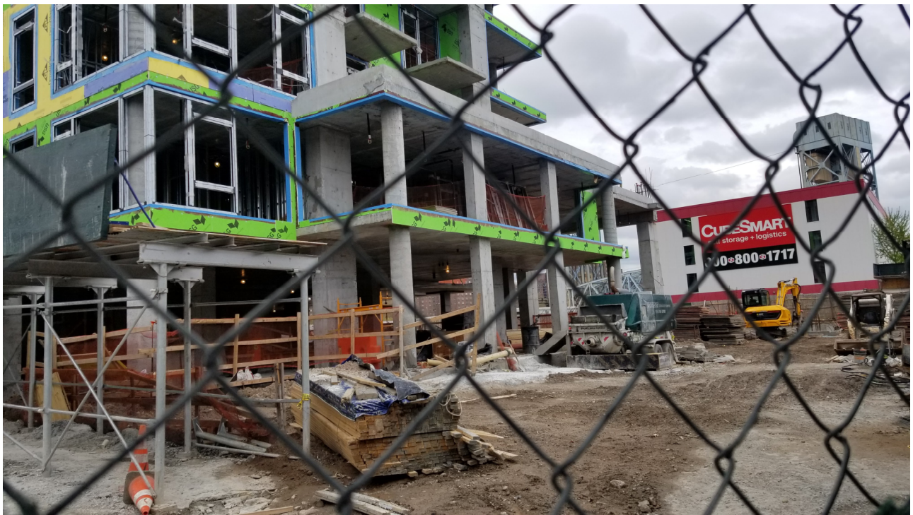
Photograph 8: View of western adjoining property (198 East 135 th Street), facing north.
