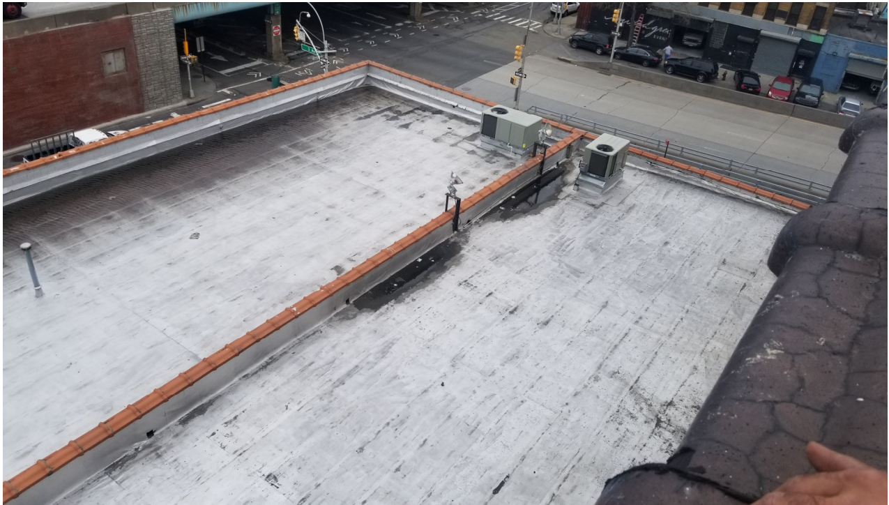
Photograph19: General view of building supply store rooftop, facing southeast.
