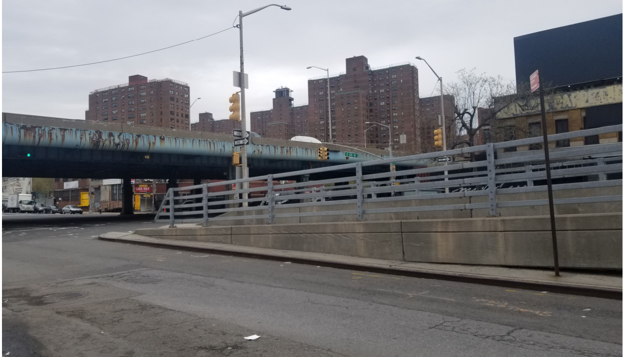
Photograph 5: View of the eastern adjoining Third Avenue and Third Avenue Bridge ramp, facing southeast.
