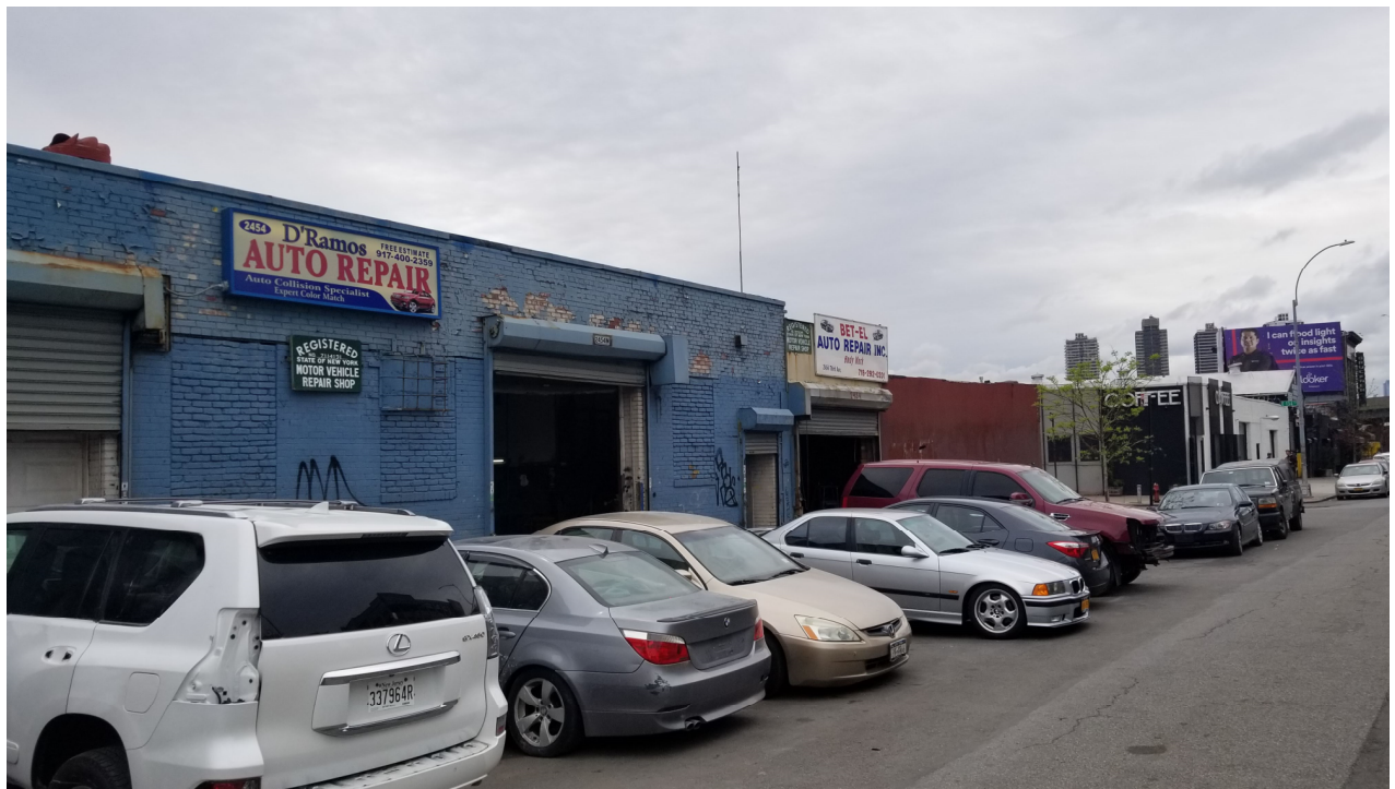
Photograph 4: View of the southeastern adjoining properties across Third Avenue, facing southwest.
